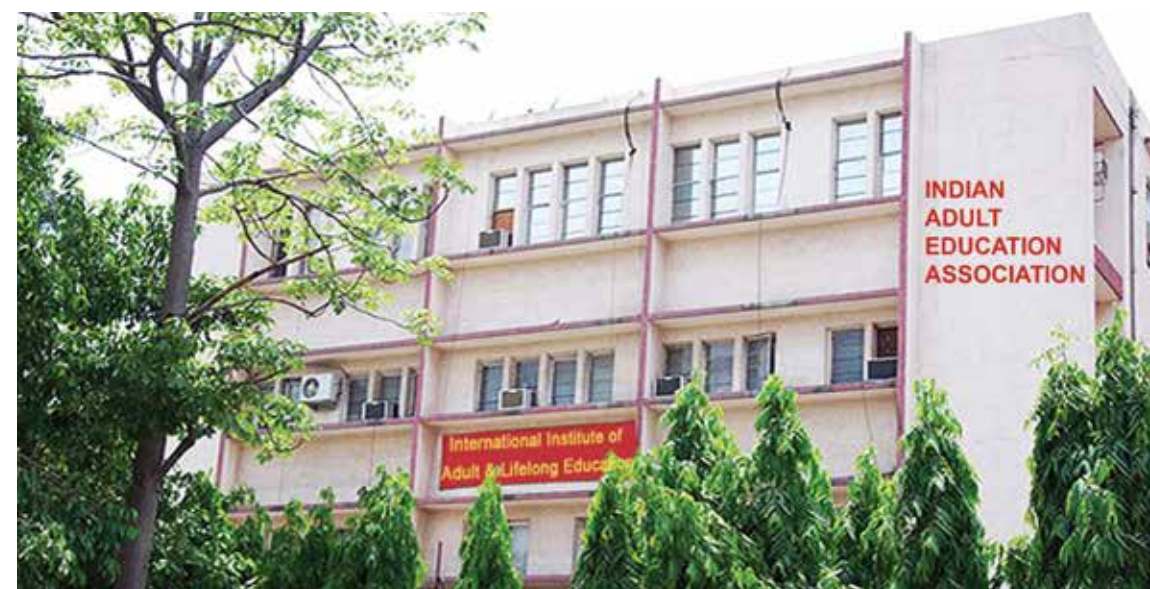
IAEA Building as on March, 2018
